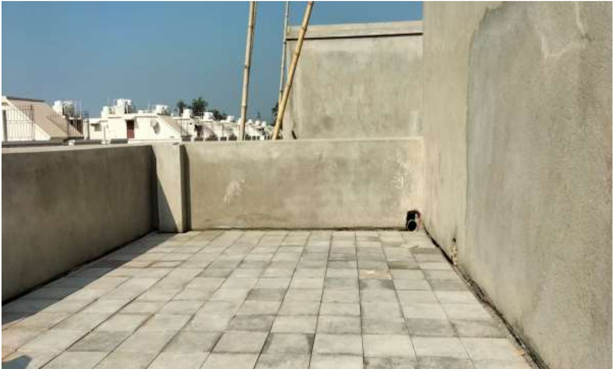
Roof Tiles work at E1
